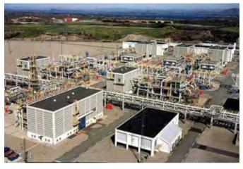
compression does not require the use of any of the natural gas from the pipe; however it does require a reliable source of electricity nearby. The compression includes a large section of associated equipment such as scrubbers (to remove liquid droplets) and heat exchangers, lube oil treatment etc.
