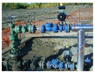
hole with casing, evaluating the pressure and temperature of the formation, and then installing the proper equipment to ensure an efficient flow of natural gas from the well. The well flow is controlled with a choke.
