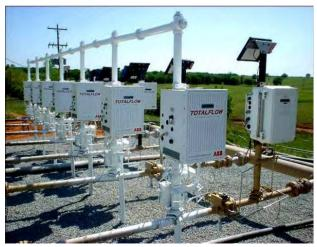
allow set up of production "well sets" so that for a given production level, the best reservoir utilization, well flow composition (gas, oil, waster) etc. can be selected from the available wells.
