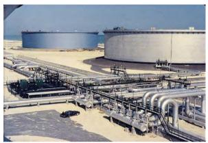
allow a shuttle tanker to offload about once a week. A larger production complex generally has an associated tank farm terminal allowing the storage of different grades of crude to take up changes in demand, delays in transport etc.
